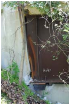
Figure 6 Shift of Superstructure (Tawarayama Bridge)
