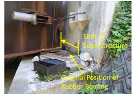
Figure 5 Shift of Superstructure (Okirihata Bridge)
