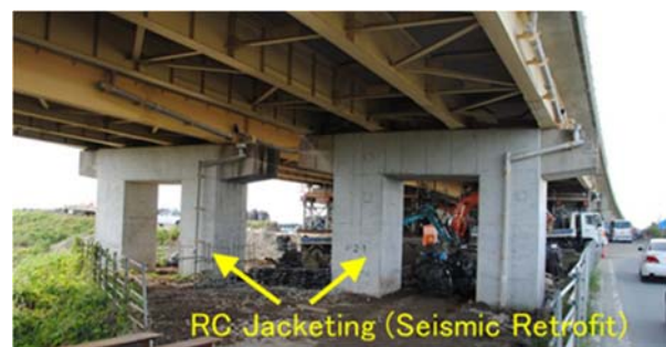
Figure 2 Seismic Retrofit of Columns (Kiyamagawa Bridge)
