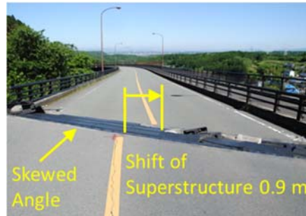
Figure 4 Shift of Superstructure (Okirihata Bridge)
