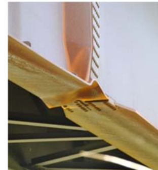
Figure 8 Shift of Superstructure (Tawarayama Bridge)
